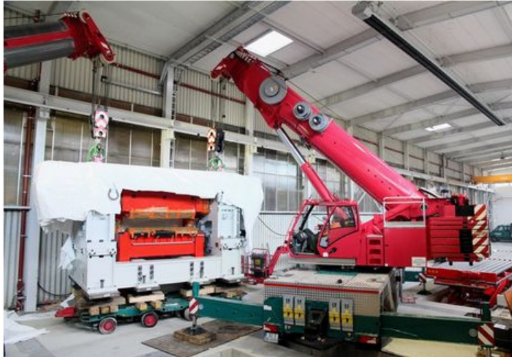
The two Grove GMK4100S carrying out their first lifts together
